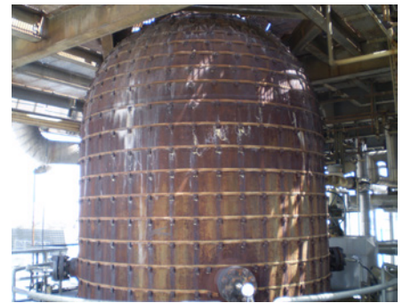
Gasifier without thermal imaging
